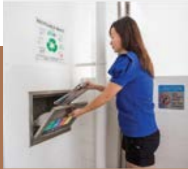
SEPARATE CHUTES FOR RECYCLABLE WASTE
