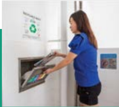
SEPARATE CHUTES FOR RECYCLABLE WASTE
